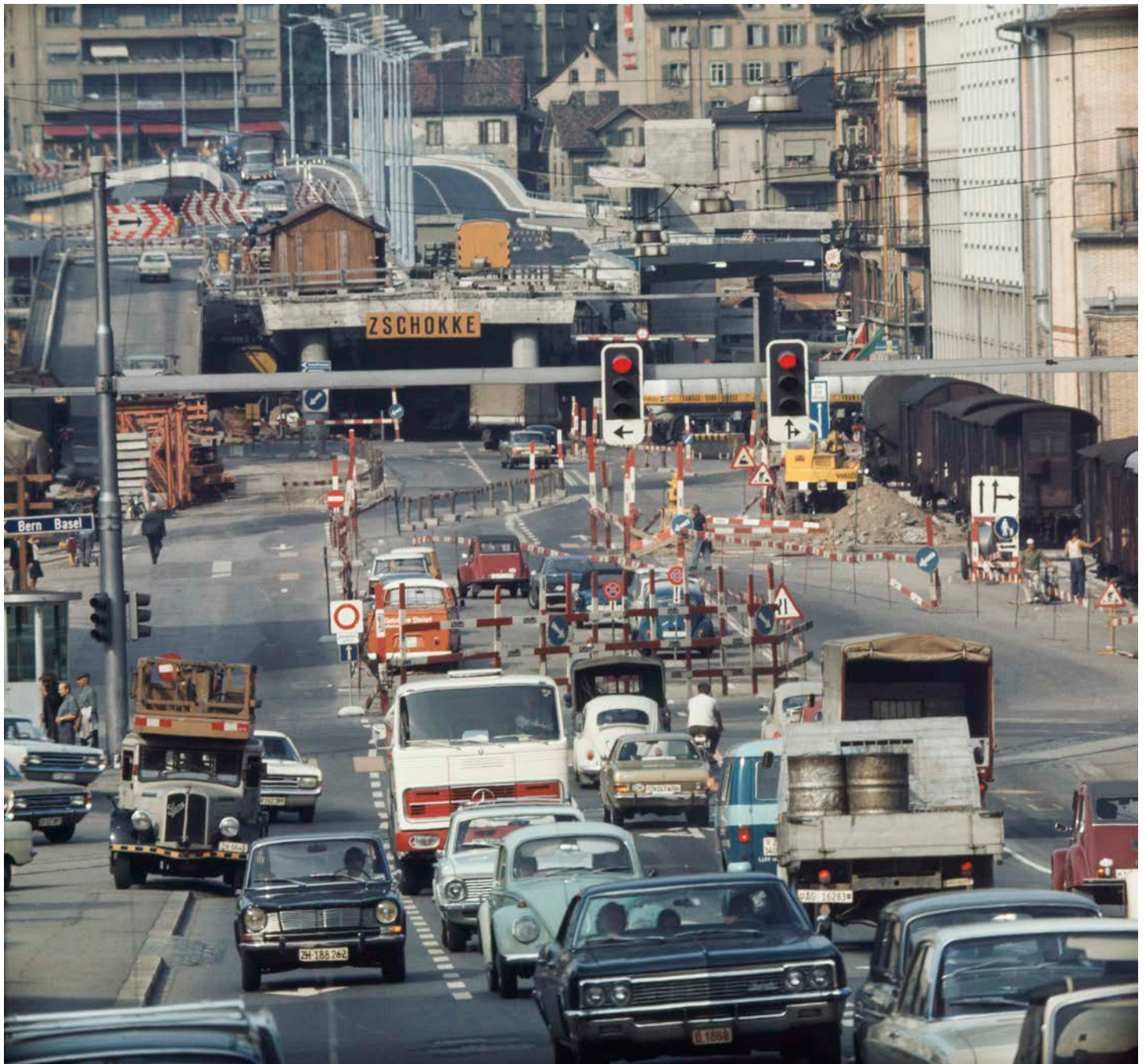
COMET PHOTO AG, CONSTRUCTION OF HARDBRÜCKE (1970)
