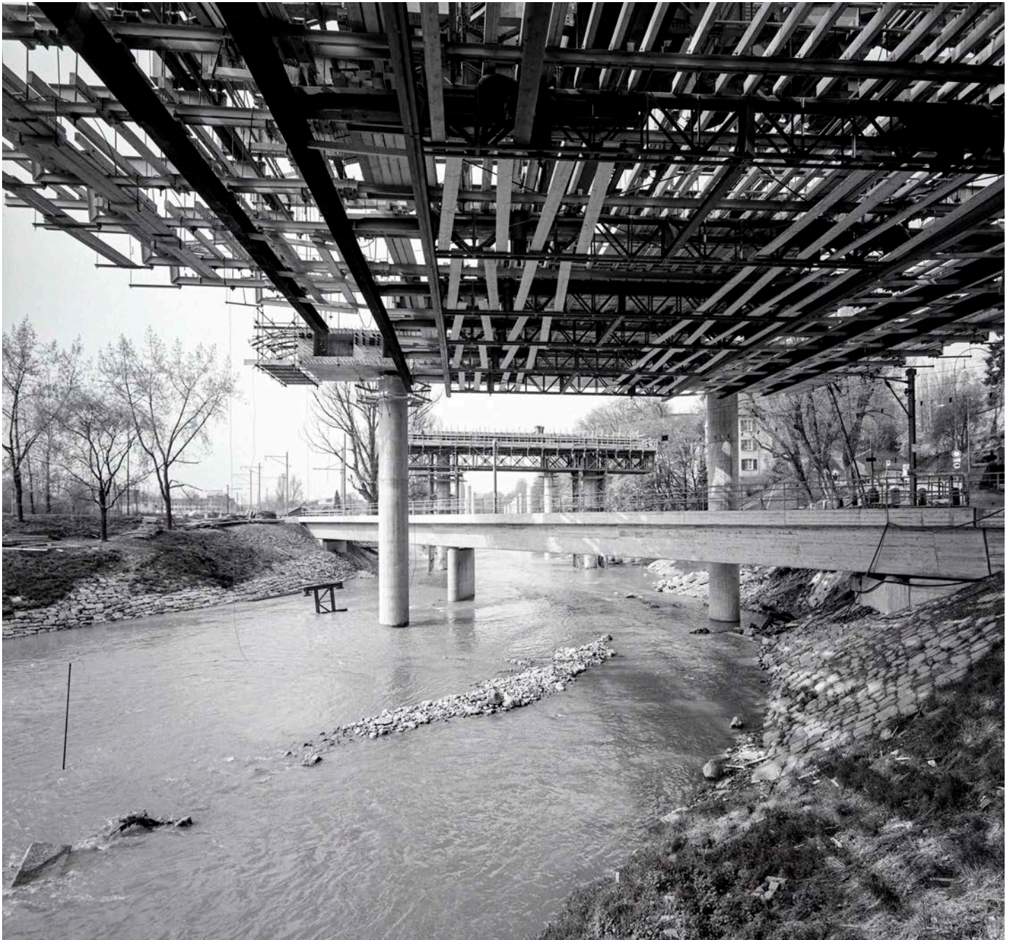
MICHAEL WOLGENSINGER, SIHLHOCHSTRASSE DURING CONSTRUCTION (1969-73)
